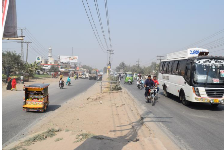
Figure 1-2: Existing Traffic Pattern on National Highways
